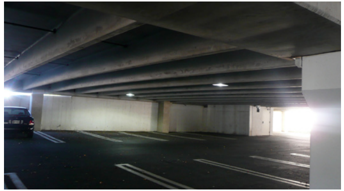
Figure 8(c). Photo – corner of parking structure
