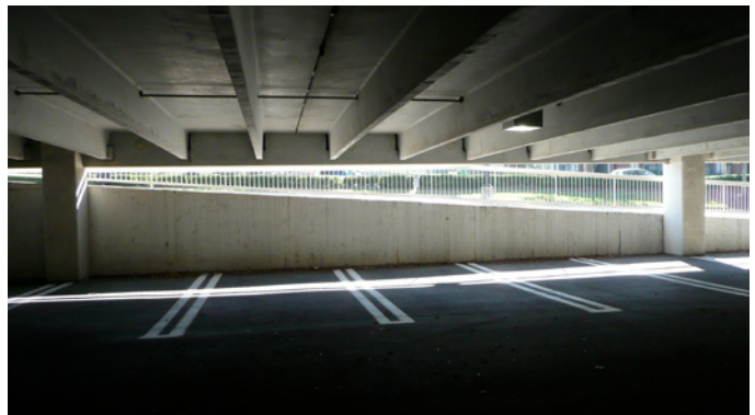
Figure 8(d). Photo – typical ceiling construction
