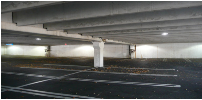
Figure 9(a). Photo of site
