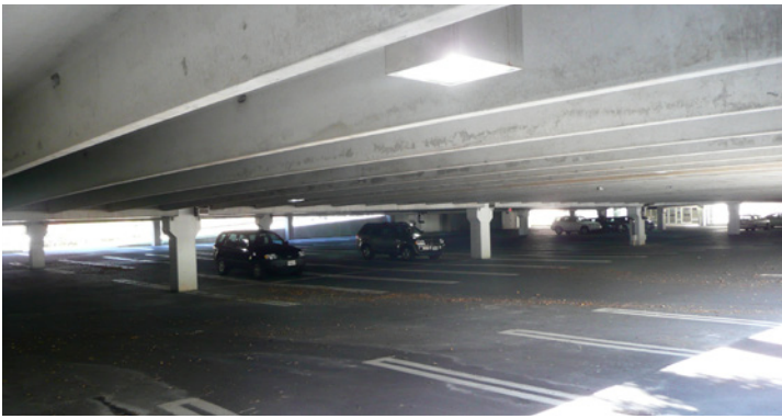
Figure 8(a). Photo – perspective of the parking structure
