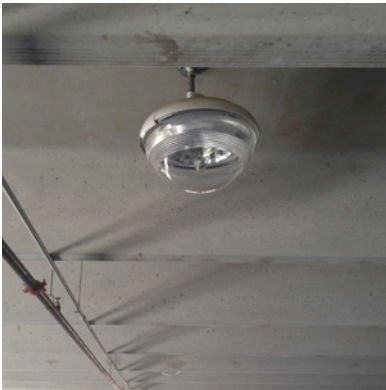
Figure 4. Corporate parking structure in Phoenix, AZ, where light is absorbed by the adjacent structural supports.
