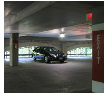
Figure 2. Tufts University incorporates daylighting into their parking structure.
