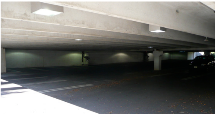
Figure 8(b). Photo – entrance during the day
