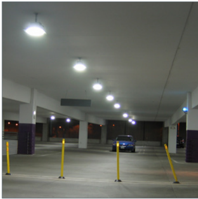
Figure 3. Arizona State University parking structure with painted white ceiling and other high reflectance materials.
