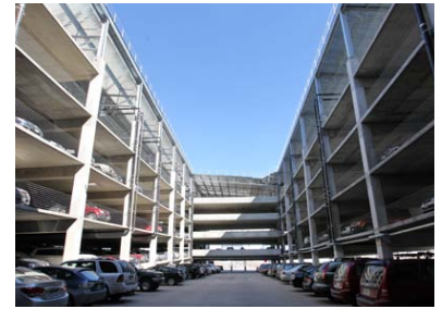
Figure 1. National Renewable Energy Laboratory’s parking structure – open building design allows for daylight design. The design of the parking structure can affect the energy performance of the structure more than luminaire selection.
